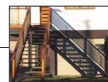
2. Wood Entry Stair
