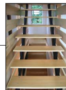
6. Wood Interior Stair
